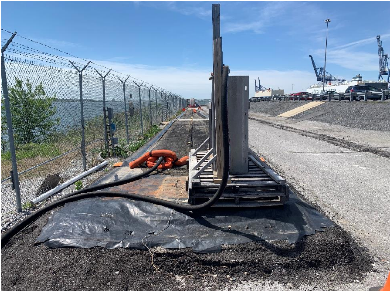
Figure 1-4 Inflow System Splitting Flow Between Two Adjacent Flow-Ways
