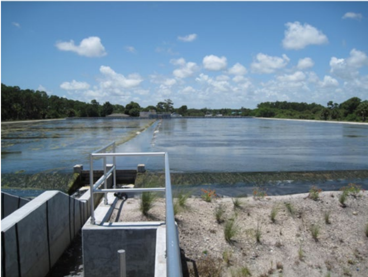
Figure 6-2 Osprey Marsh Algal Turf Scrubber™ in Indian River County, Florida
