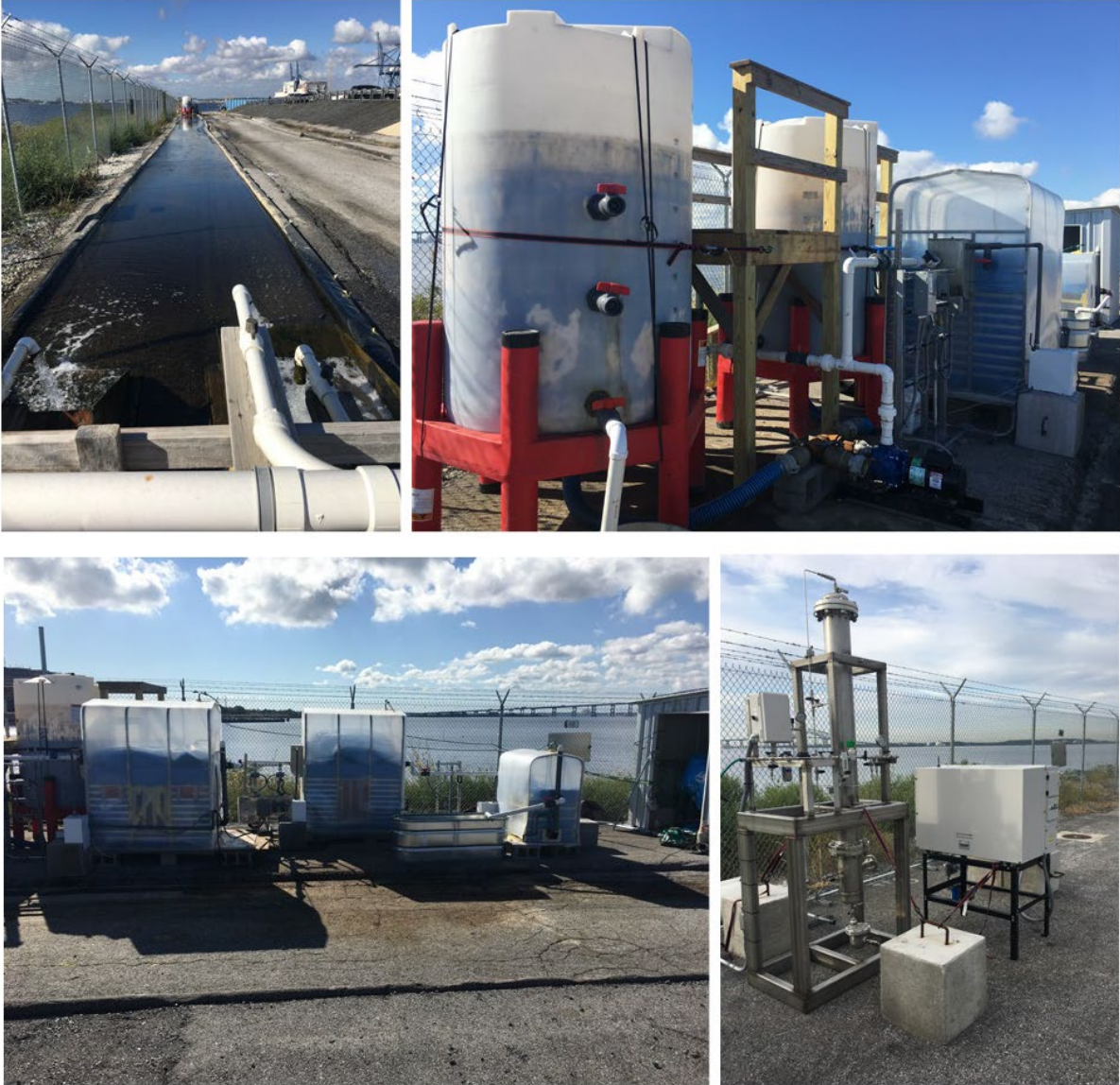
Figure 1-3 Photographs of the Components of the Integrated System
