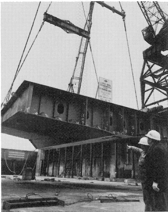
Huge cranes move keel piece into position at General Dynamics Quincy Shipbuilding Division. Laying of the 120-ton unit marked construction of the second Seabee for Lykes Bros. Steamship Co., the ALMERIA LYKES.
