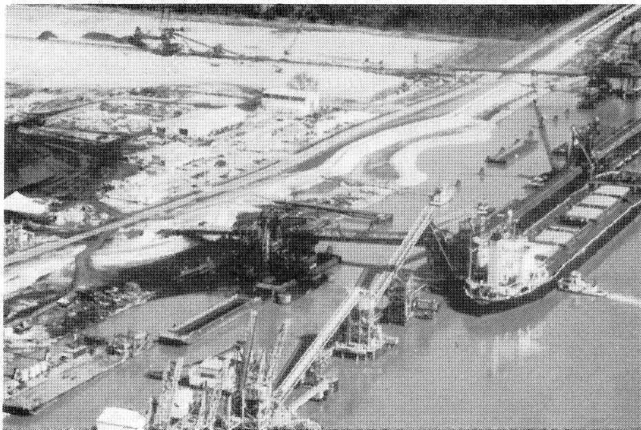
Newly expanded electro-coal transfer facility at Danville, IL, now has an annual throughput capacity of more than 25 million tons and on-ground storage capacity of 4.5 million tons of coal.
