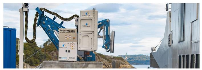
Figure 61: Wärtsilä/Cavotec DC shore charging and mooring system with 690VAC input (source: Wartsila)
