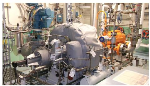
Figure 70: Curtiss-Wright steam turbine generator (source: Curtiss-Wright)
