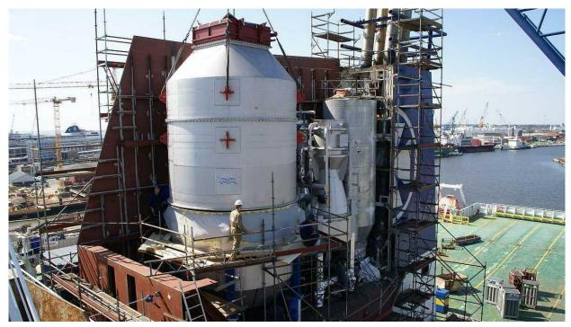
Figure 129: Alfa Laval has tested its SOx scrubber technology to absorb CO2 (source: Alfa Laval via rivieramm.com)
