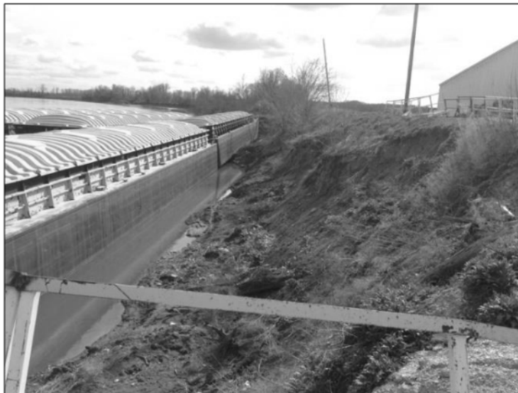
Figure 10: Existing Stationary Dock Barge – Bank Erosion
