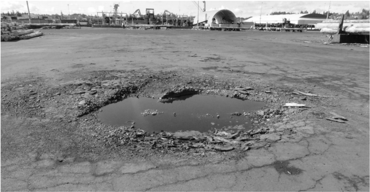
Figure 6 Ponding and localized alligator cracking is also found throughout the site
