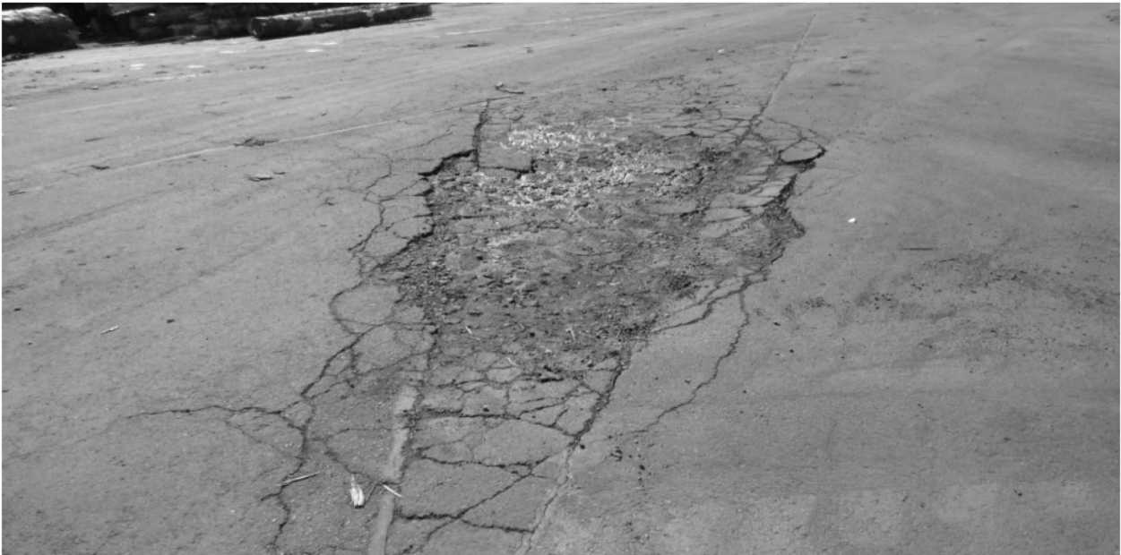
Figure 7 The patchwork done along the border between the Marine Terminal Site and the Berthing has created a raised platform that can cause damage to heavy machinery while transporting logs
