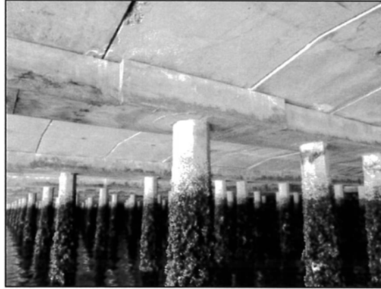
Figure 4: Pier-to-beam connection (with beam modification for as-built pier location)
