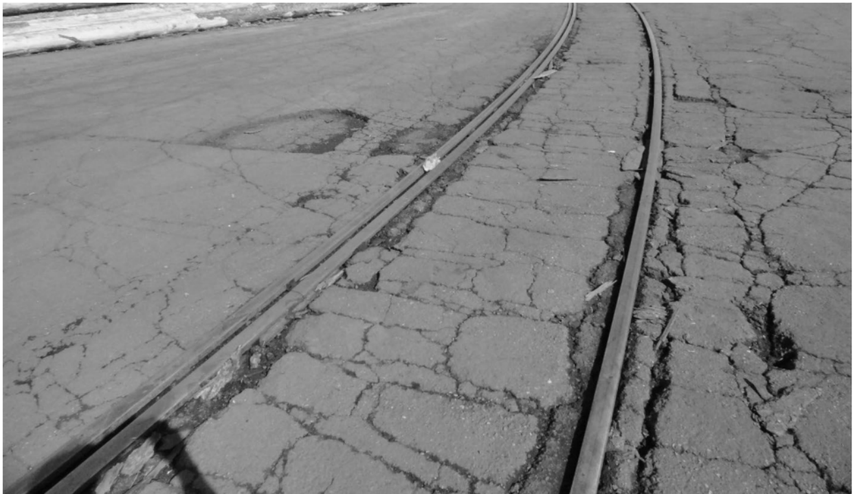
Figure 4 Localized depressions are present mostly in areas where there is constant heavy machinery traffic, including the train tracks and areas where log holders were placed
