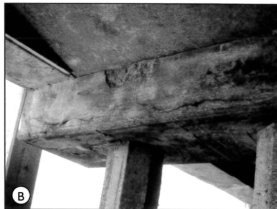
Figure 1: (A) Typical discoloration and cracking on bent cap; (B) significant cracking on bent cap.
