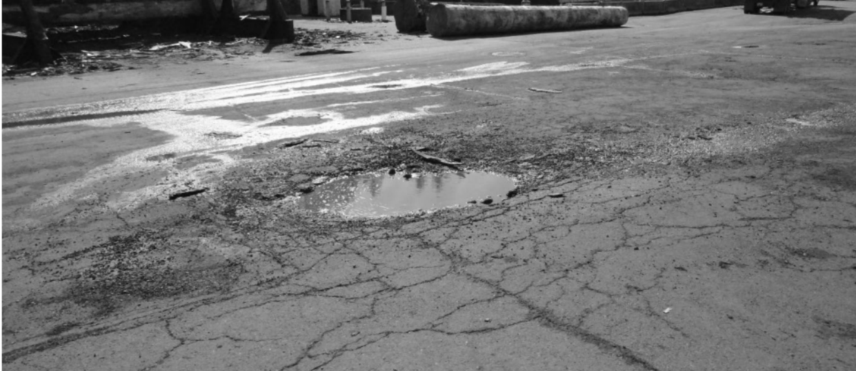
Figure 5 There is cracking around utilities and storm drainage grates as well as broken underground drainage pipe and storm vault on the northwest side of the site
