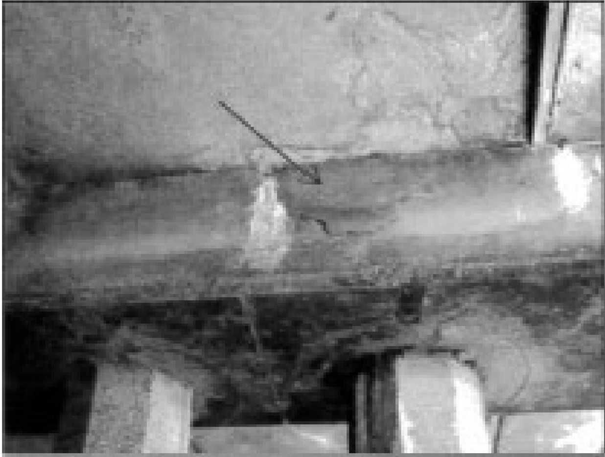
Figure 3 Spall in the inverted beam
