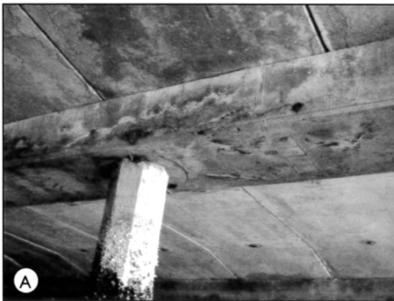
Figure 1: (A) Typical discoloration and cracking on bent cap; (B) significant cracking on bent cap.
