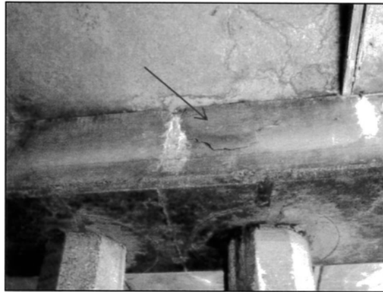
Figure 2: Spall in an inverted-T beam.
