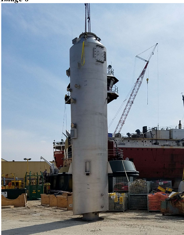
Scrubber vessel being lifted for installation
