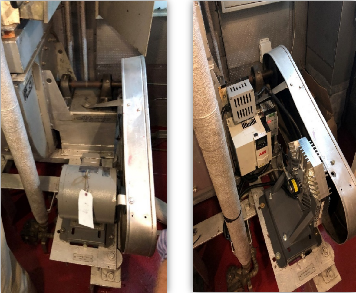
Figure 02: ECM Motor Installation Before and After
