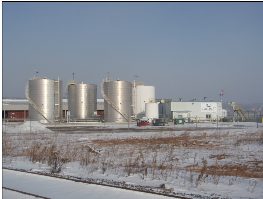
Figure 15: Calumet Superior, LLC., Duluth Marine Terminal Storage Tanks Source: Dr. Stewart, Richard
